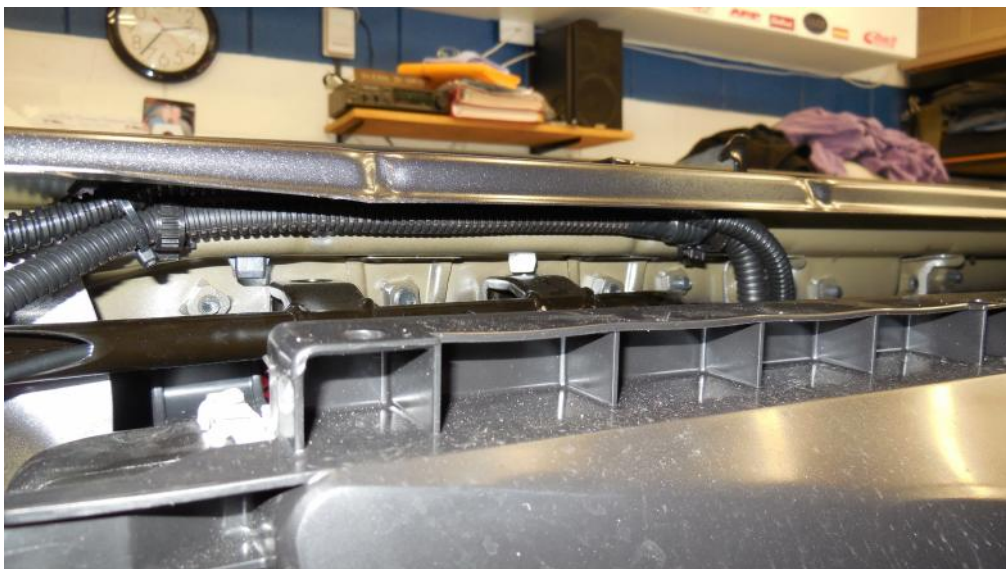
Zip tied the harness to the existing truck harness.
